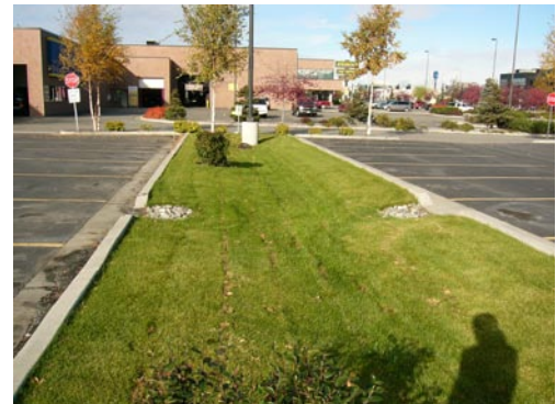
Parking Lots in Anchorage: Top shows curb cuts with flow to filter strip, bottom shows curb cuts with infiltration areas
