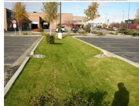
Top: Roof drainage to planter in Portland Bottom: Infiltration trench in Anchorage
