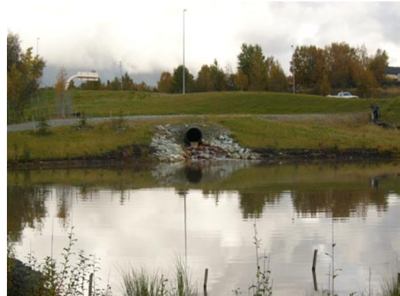
Inlet and Sediment Forebay in Anchorage
