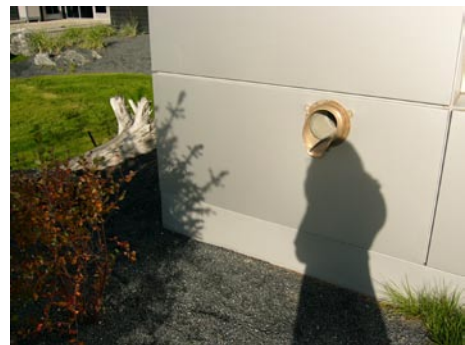
Roof downspout into planted infiltration area
