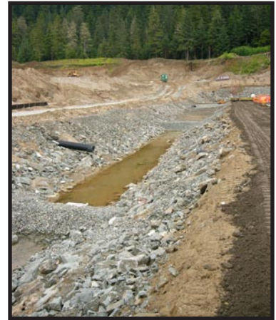
Sand Filter during construction of Home Depot, Juneau
